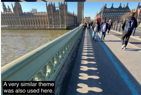
This bridge was designed to have shadows that reflect the pianists who work nearby.
